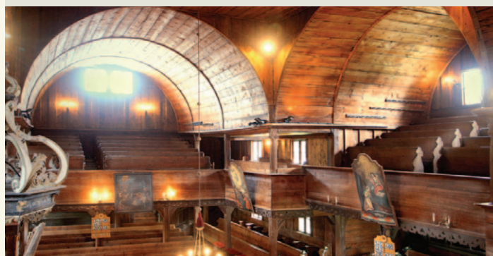
▲ Drevená stĺpková architektúra a valená dosková klenba – Hronsek Wooden columnar architecture and planked barrel vaults of the Lutheran church in Hronsek
